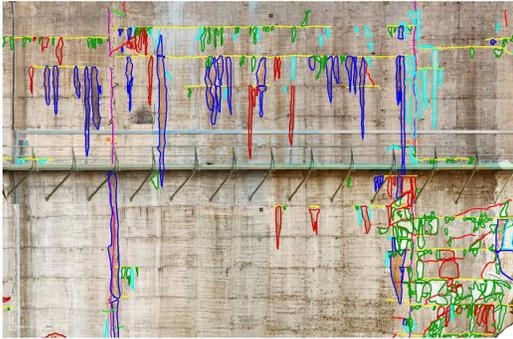
Figure 2 - Ortoimages as a base map for heads up vectorisation of anomalies classified and symbolised according to a catalogue.
