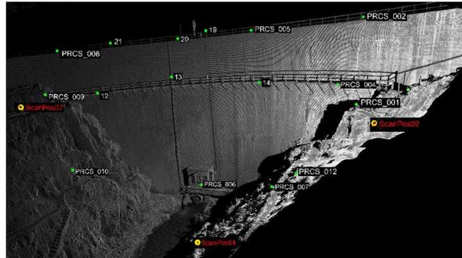
Figure 1 - A perspective of the laser intensity 3D model of Alto Ceira dam downstream face, layout of stations (with red labels) and retro-reflector targets (with white labels).
