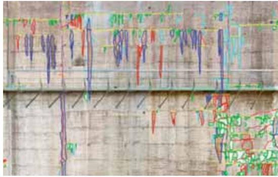
Figure 2: Orthoimages used as a base map for vectorisation of the anomalies classified according to a catalogue.
